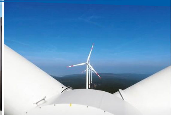
© Vensys 112, 2,5 MW, Wind farm in Losheim-Britten, Germany
