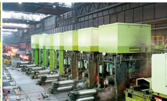
© ThyssenKrupp AG RS32572
